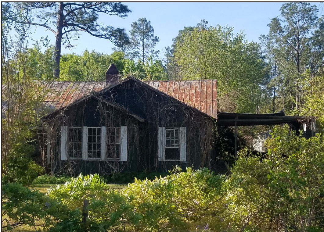
Figure 25. View of HS3, looking south from SR94.
