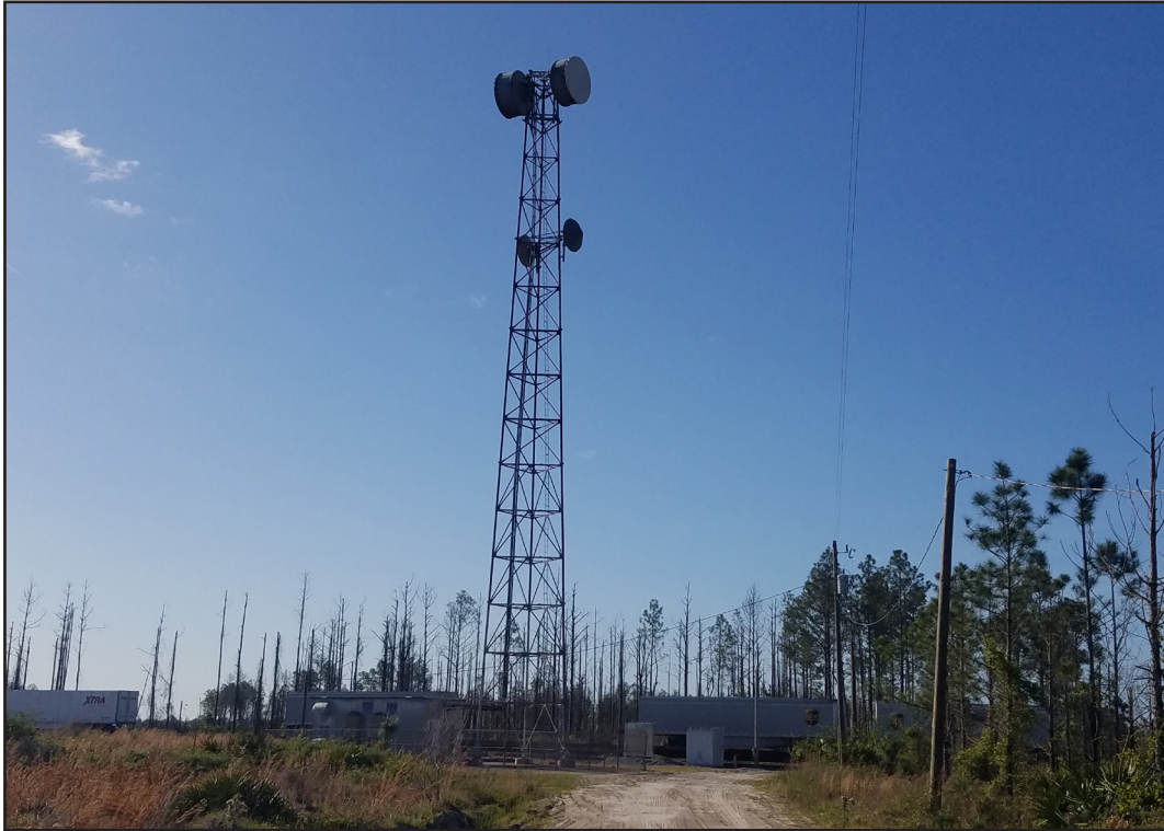
Figure 24. View of HS1, looking south from SR94.
