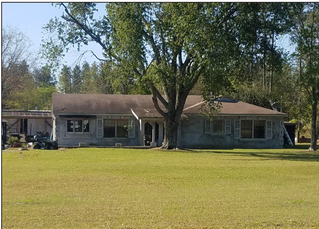
Figure 27. View of HS5, looking south from SR94.
