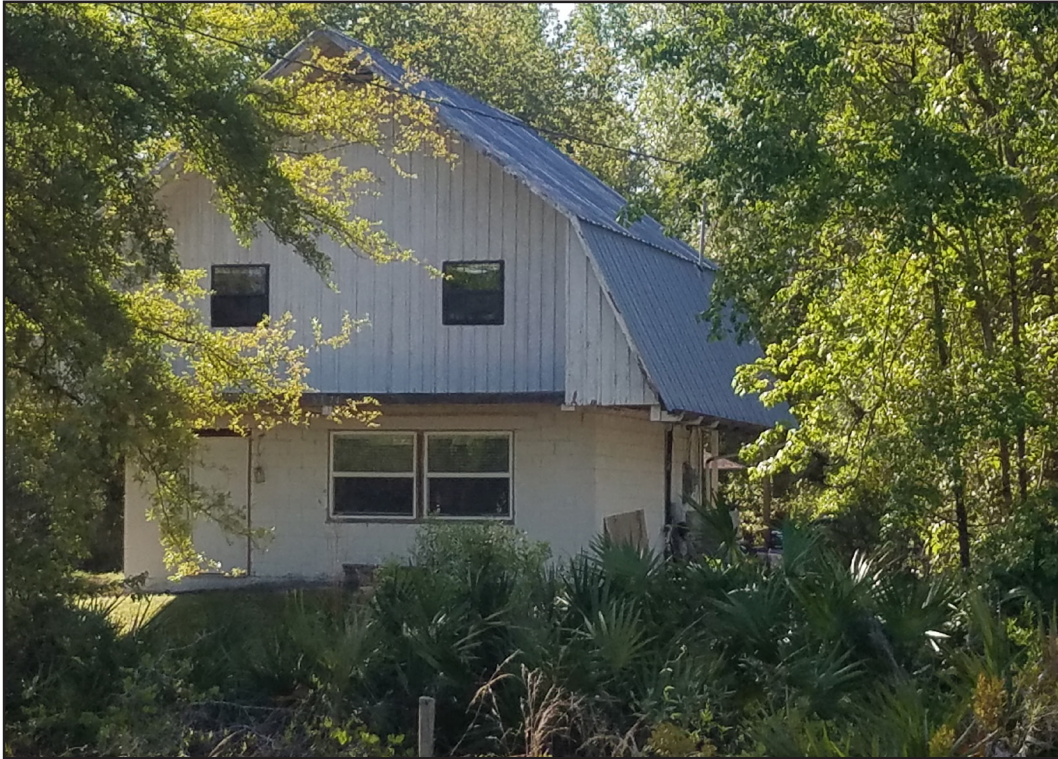
Figure 28. View of HS6, looking south from SR94.
