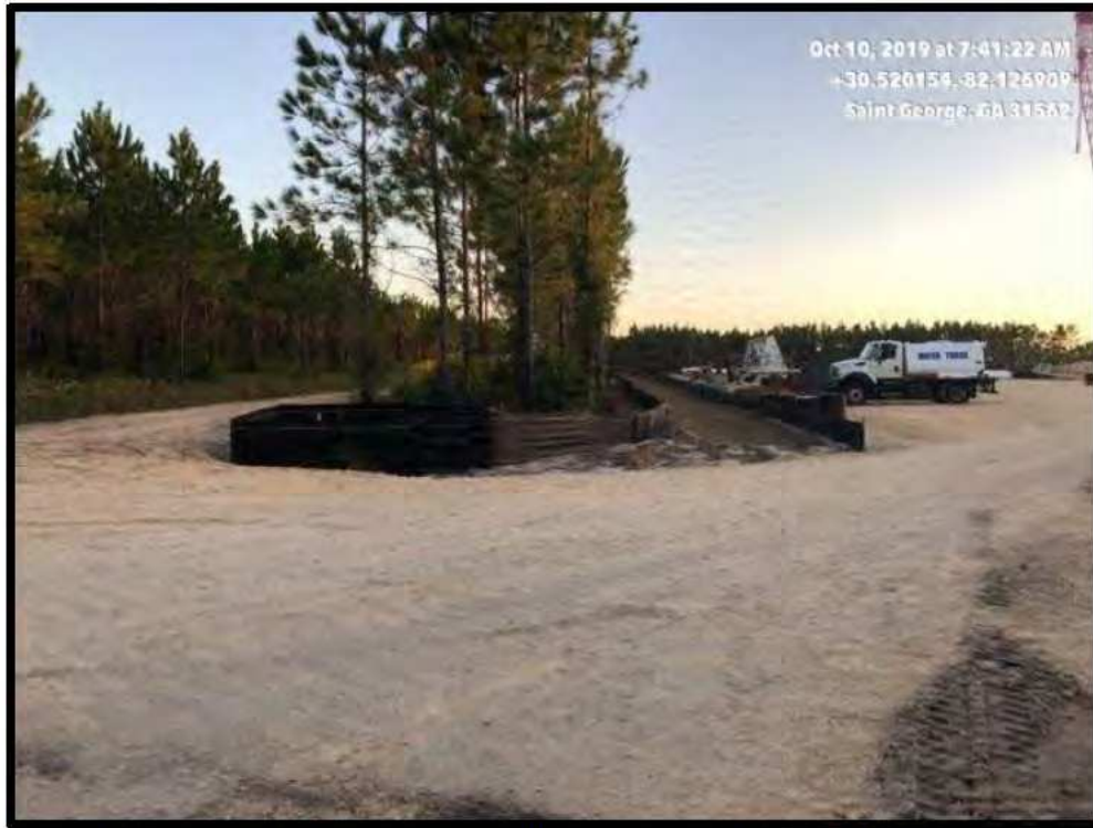
Photograph 1: View to the north of the entrance into the construction yard.
