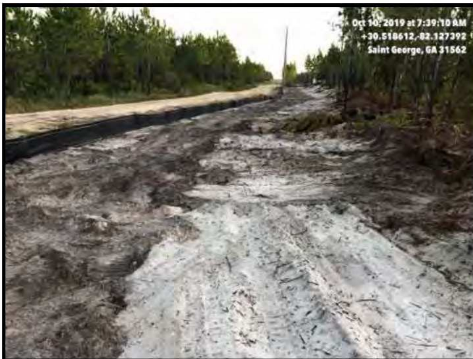
Photograph 4: View to the north of T-Model Road, silt fence, and cleared vegetation.
