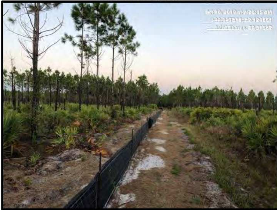
Photograph 3: View to the west of the vegetative buffer (left side of photograph) and northernmost silt fence.
