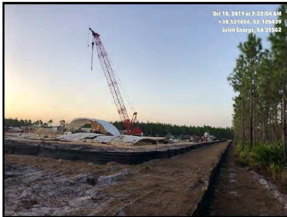
Photograph 6: View to the south of the construction yard with BMPs.
