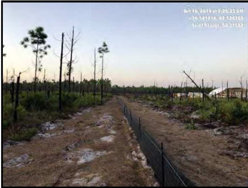
Photograph 5: View to the west of the vegetative buffer (right side of photograph) and northernmost silt fence.
