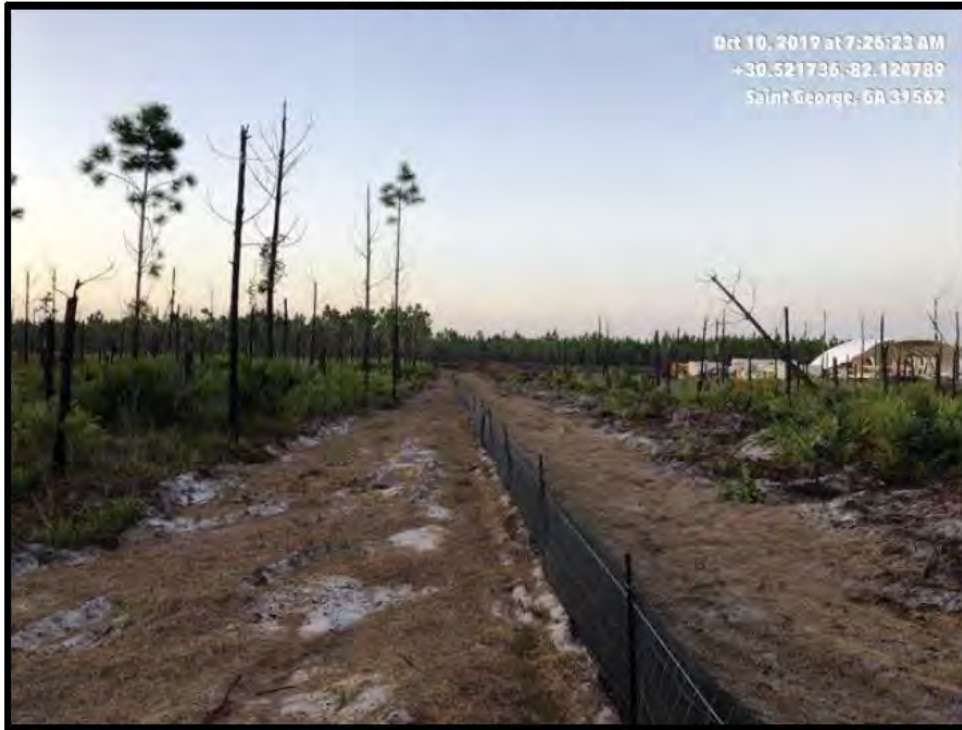
Photograph 5: View to the west of the vegetative buffer (right side of photograph) and northernmost silt fence.
