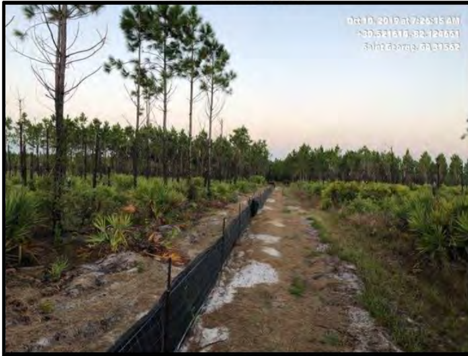
Photograph 3: View to the west of the vegetative buffer (left side of photograph) and northernmost silt fence.
