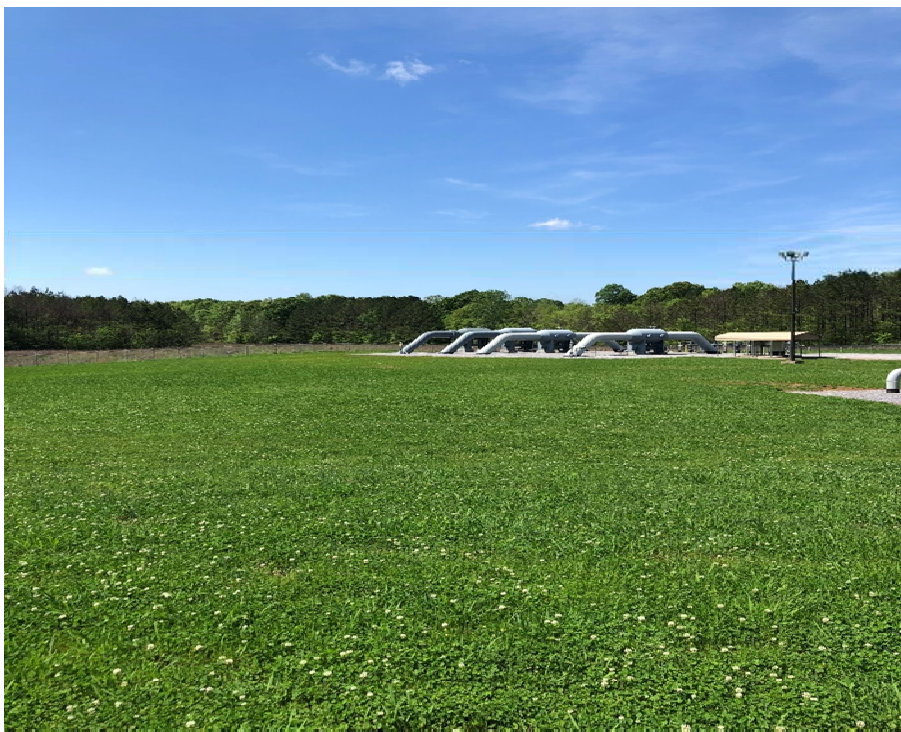
Photo 18: Station 95. View of restored temporary workspaces around the scrubbers on 3/25/2020. Facing northwest.
