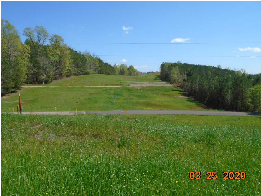
Photo 13: Verbena Loop. View of restored right- of-way around the County Road 519 and 520 crossings. Facing east.
