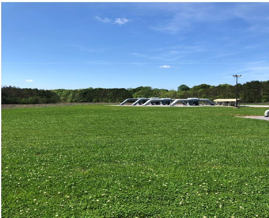
Photo 18: Station 95. View of restored temporary workspaces around the scrubbers on 3/25/2020. Facing northwest.
