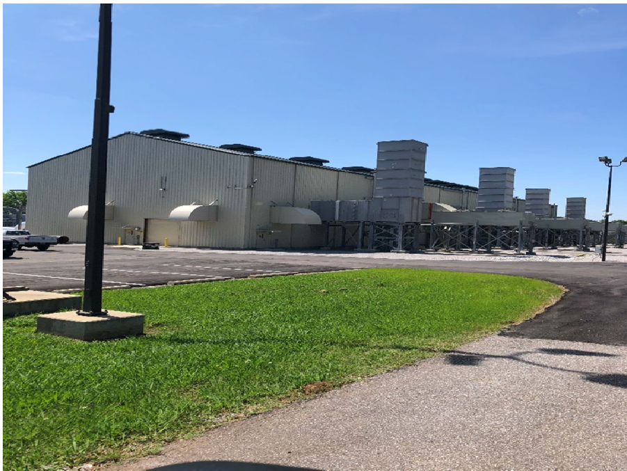
Photo 16: Station 95. View of the new addition on the east side of the facility on 3/25/2020. Facing south.
