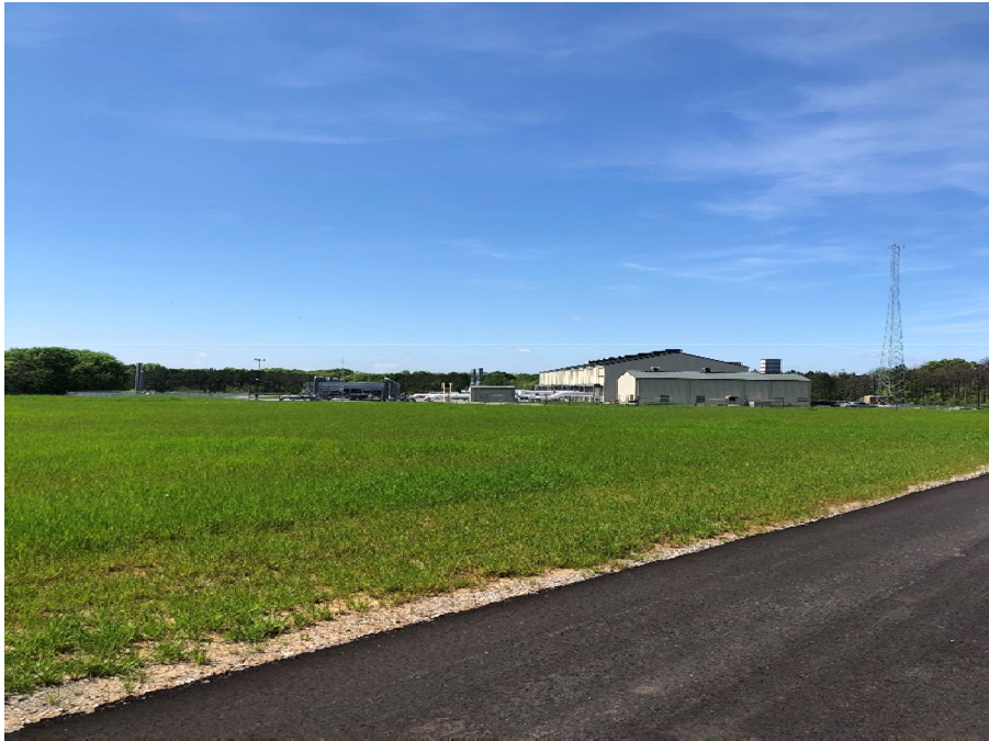
Photo 15: Station 95. View of restored temporary workspace north of the facility entrance road on 3/25/2020. Facing west.
