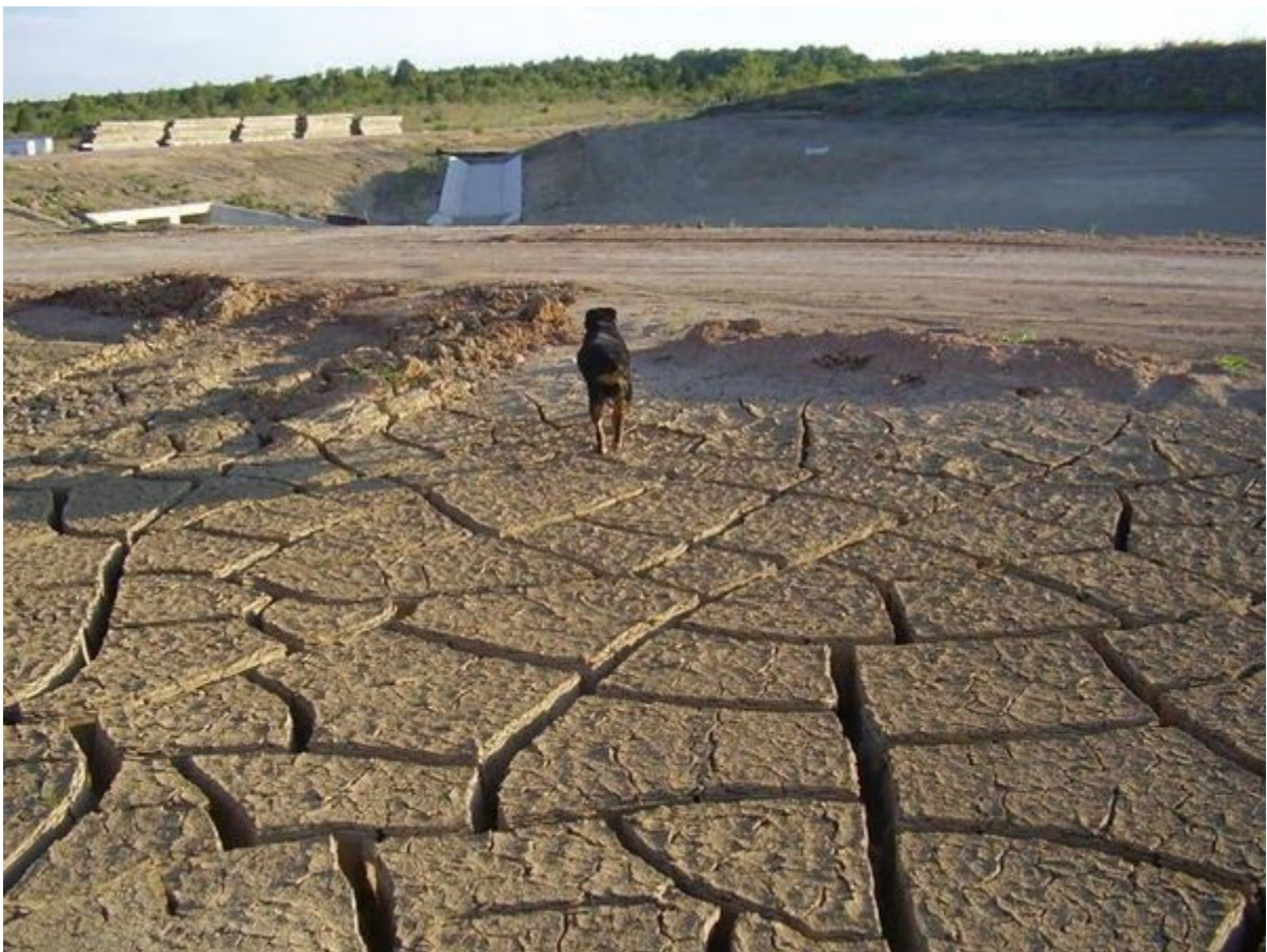
Photo: Gretchen Quarterman, Cracked dirt and SH 130 construction , 2006-08-11.
