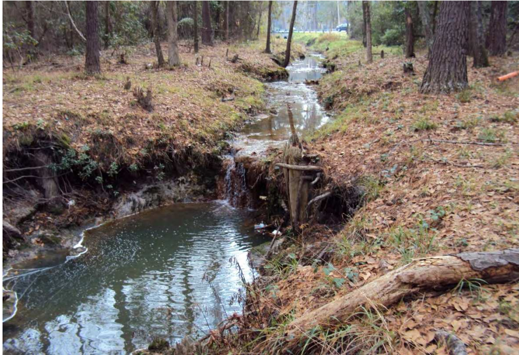
Figure 3.3.4. Knick Point 250 feet Downstream of River Street
