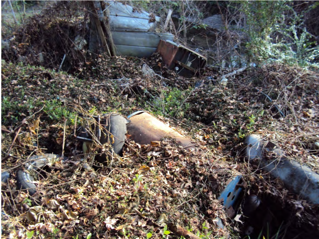
Figure 3.3.10. Gullies Filled with Garbage and Debris Downstream of W. Magnolia St.
