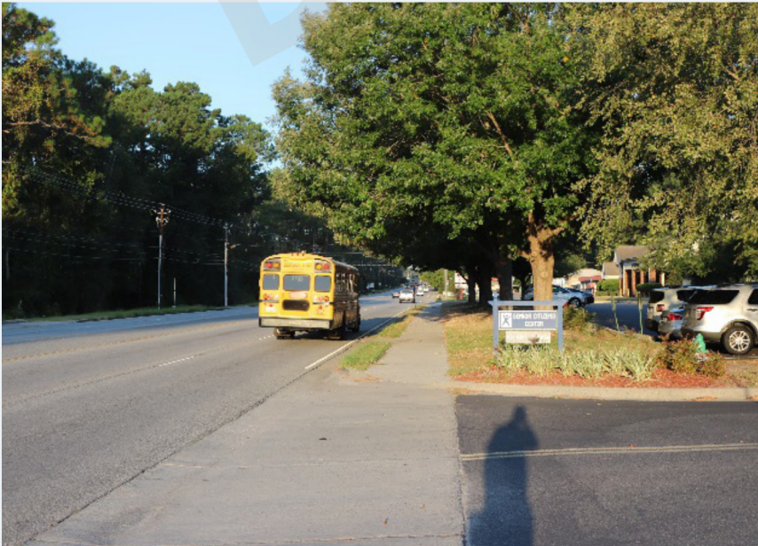
Sidewalks along the Senior Center with limited buffer and separation from fast moving traffic
