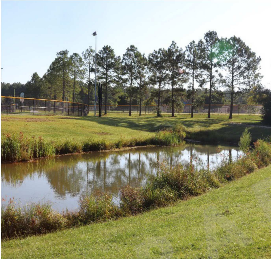
Example of wet-retention pond with littoral and pond bank vegetation at Freedom Park
