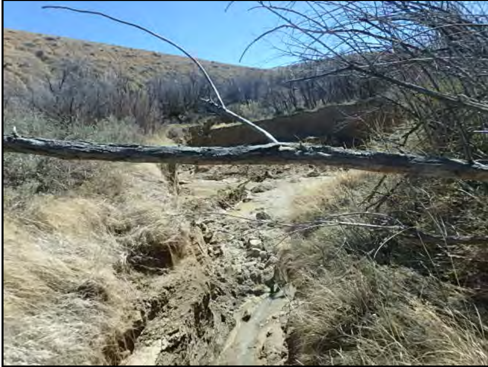
Photograph B-3. Meyer Draw where head-cutting starts just below north road crossing.
