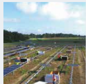
Rack & Module Installation
