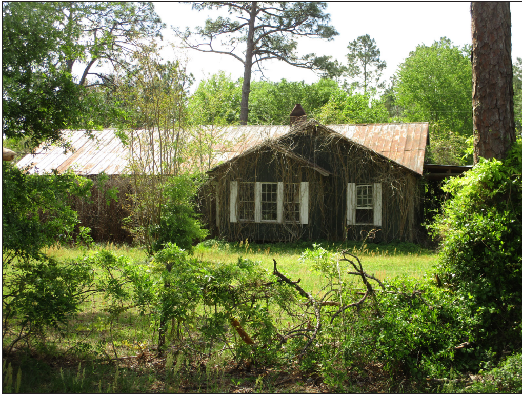
Figure 24. View of the house located at 8208 SR 94, facing south.
