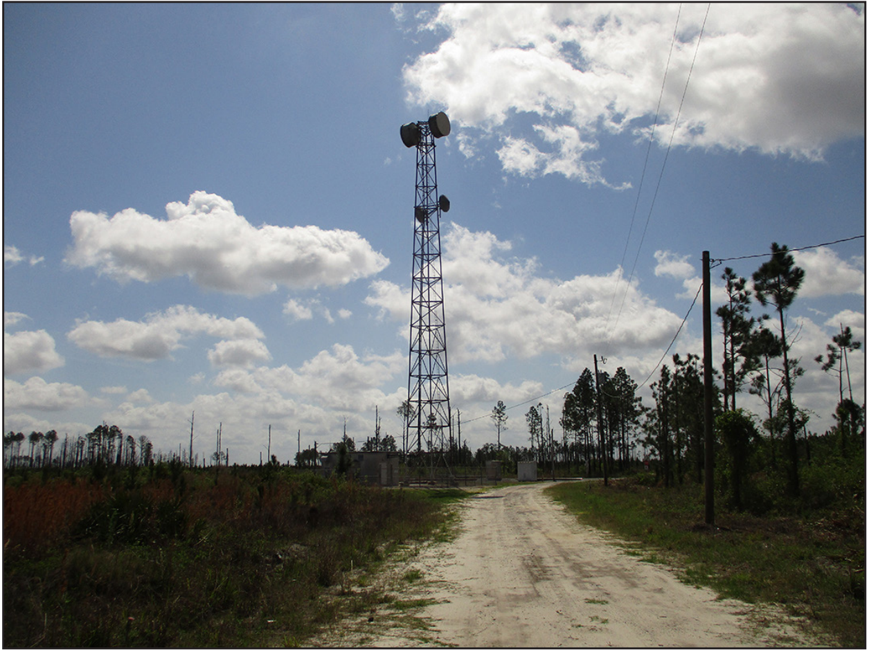
Figure 59. View of radio tower, facing southeast.
