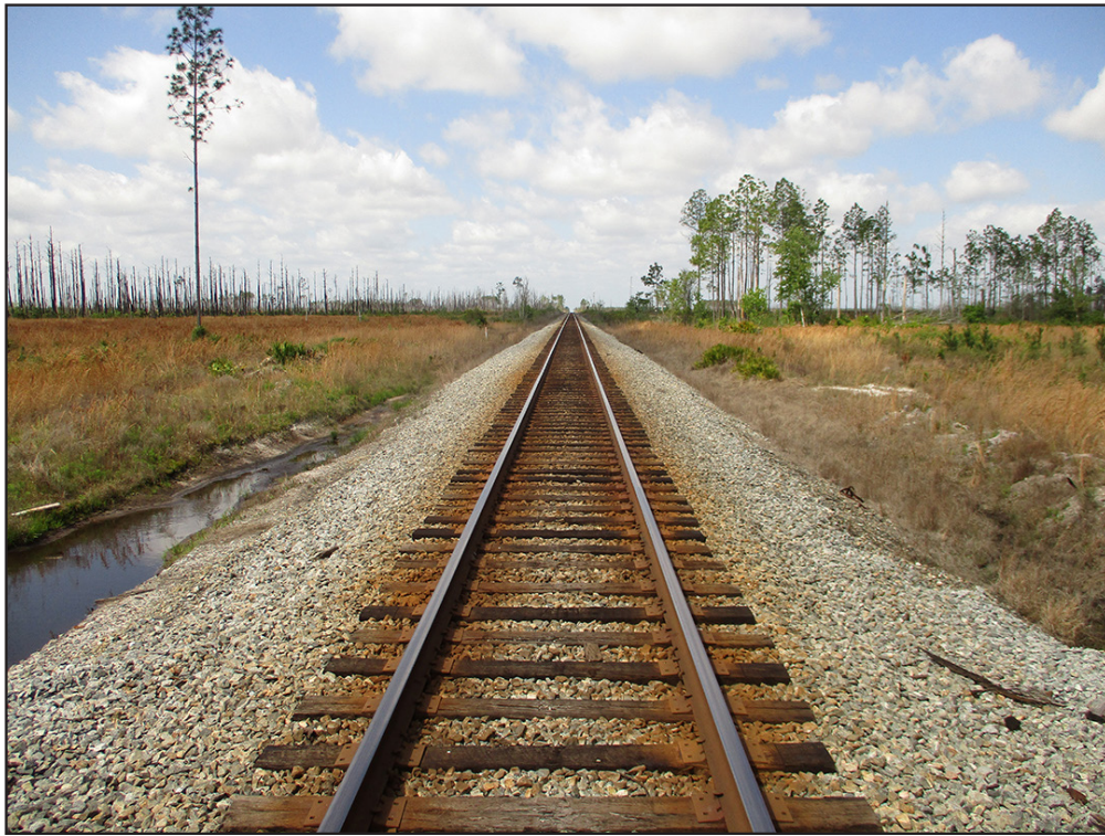
Figure 57. View of Georgia Southern and Florida Railway, facing west.
