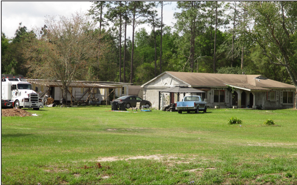
Figure 25. View of the non-historic house and trailer located at 8296 SR 94, facing southwest.
