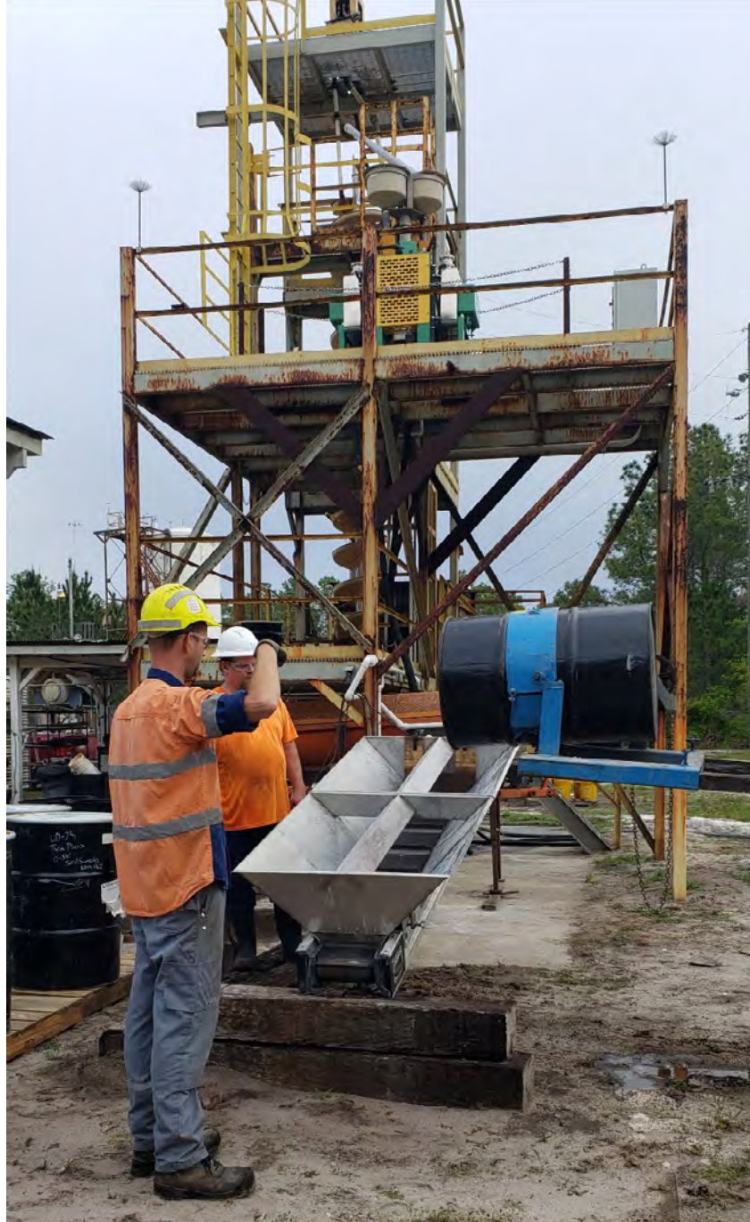
Photograph 1. Processing of UD boring drummed soil through mineral extraction processing plant.
