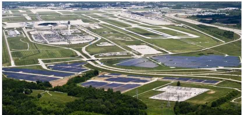
Figure 7. 20 MW PV System at Indianapolis International Airport (Photo source: inhabitat.com)
