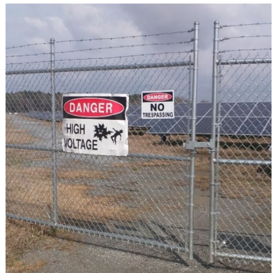
Figure 1. Perimeter Fence with Warning Signs
