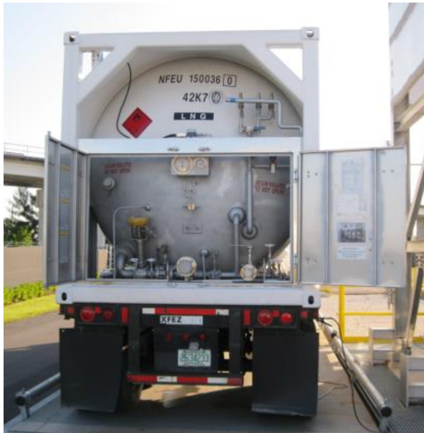
Figure 6. View of valves and outer tank penetrations inside valve cabinet.
