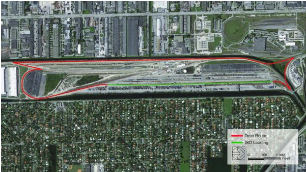
Figure 32. Aerial view of the Hialeah Yard. The train route through the yard is red and the range of lifting operations along the intermodal ramp is shown as a green line.
