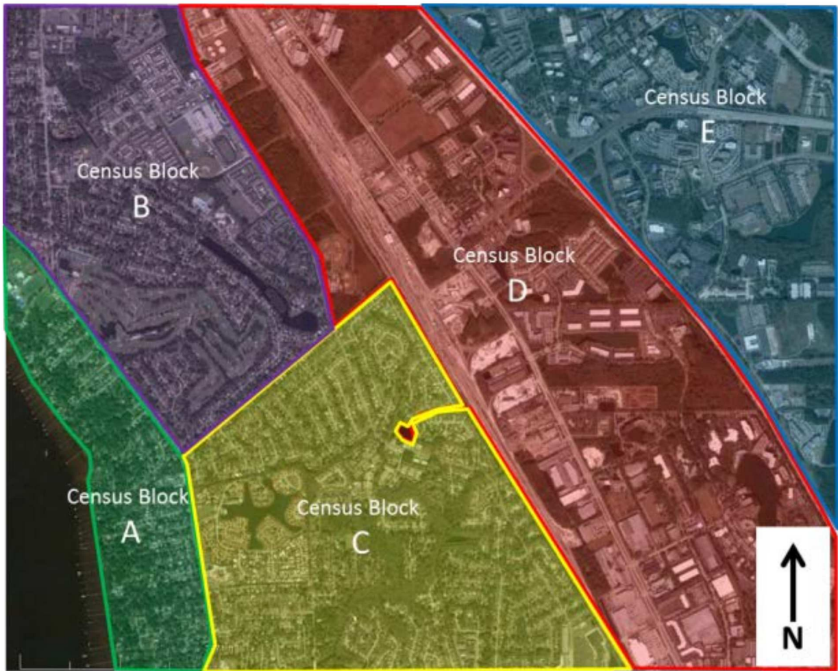
Figure 39. Aerial view of the Bowden Yard depicting the five consolidated census blocks used to represent nearby populations.
