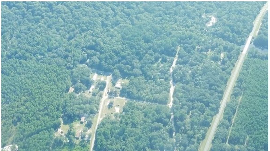
E down SE 54th St, CR 231 New River bridge, Howard mine site on right, 09:54:45, 29.9537460, -82.3515830
