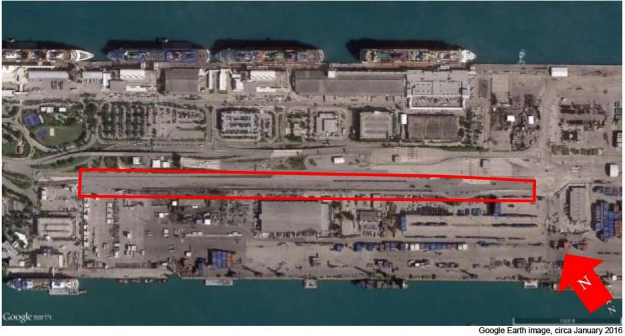
Figure 13. FECR Port of Miami Intermodal Facility (enclosed in red outline) intermodal ramps.
