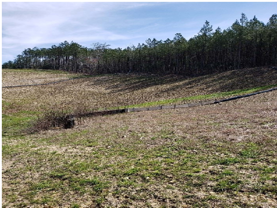
Photo 2: Rock Springs Loop. View of restored right-of-way around the WCW9C003 wetland crossing on 3/7/2020. Facing east.
