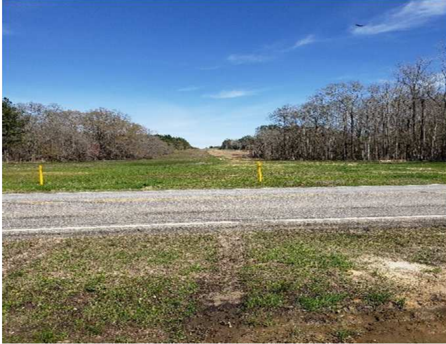
Photo 7: Rock Springs Loop. View of restored right-of-way around the Riderwood Road crossing on 3/7/2020. Facing east.
