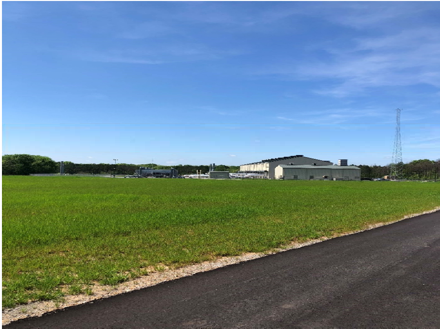
Photo 15: Station 95. View of restored temporary workspace north of the facility entrance road on 3/25/2020. Facing west.
