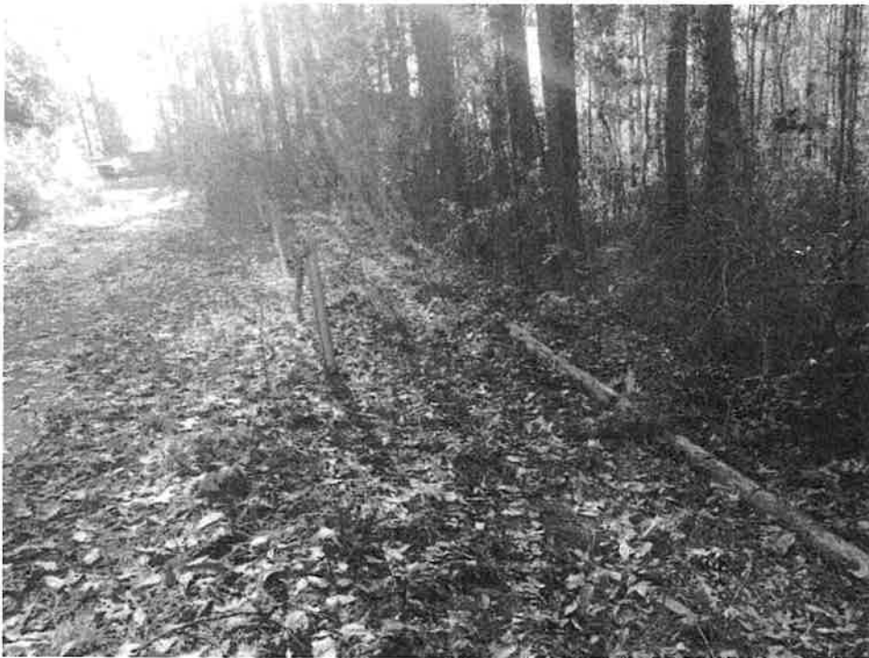
Photos 7 & 8: View of ATV access around both ends of the chain fence present along the southwest side of the dam access road, adjacent to the ATV trail shown in Photo 6. An additional section of fence will be installed to connect the fence along the entire length of the road. Additional signage will be placed in this location.
