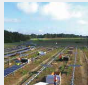
Rack & Module Installation
