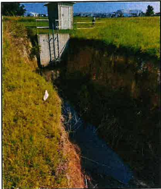
Photograph 1: Upper reach of D-1.
