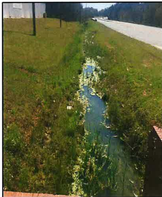
Photograph 7: View of lower reach of D-1. Photograph taken facing south.
