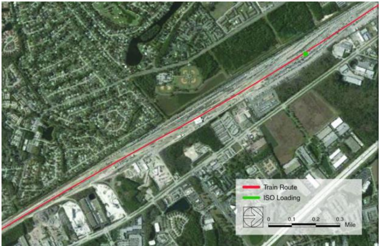
Figure 35. Aerial view of the Bowden Yard. The yard rail line is red and the approximate location of the lifting operations is represented as a green dot.
