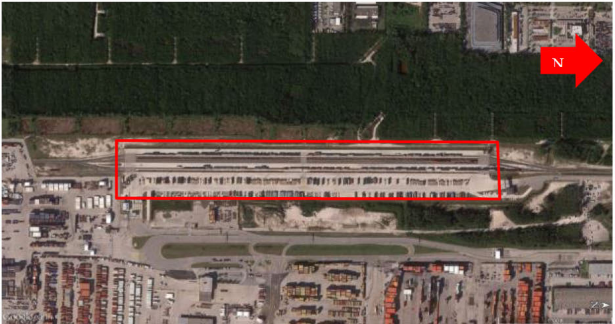
Figure 15. FECR Port Everglades Intermodal Facility (enclosed in red outline) intermodal ramps and container staging area.
