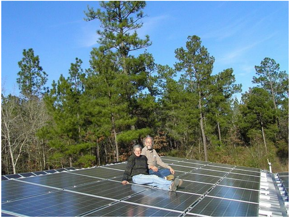
Gretchen Quarterman and John S. Quarterman on the new panels on the roof of the farm workshop at Okra Paradise Farms, Lowndes County, Georgia, 29 January 2012.
